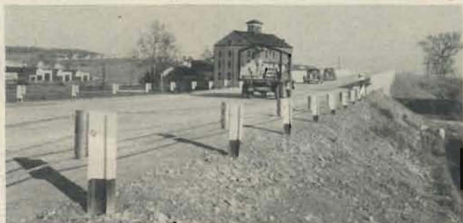
Bethlehem Cable Guard Rail, mounted on Bethlehem Steel Posts at bridge approach, affords constant protection to motorists using the new highway.
